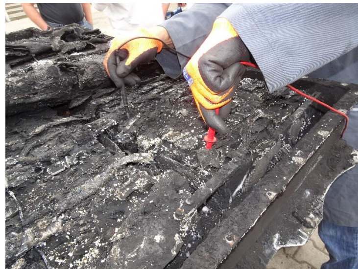
Thermal runaway in Lithium-ion hoog voltage batterij
